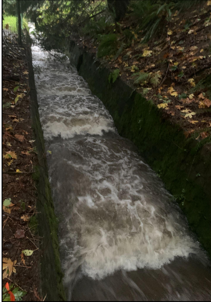
Concrete flume in Bon Accord Creek after installation of Flexi Baffles.
