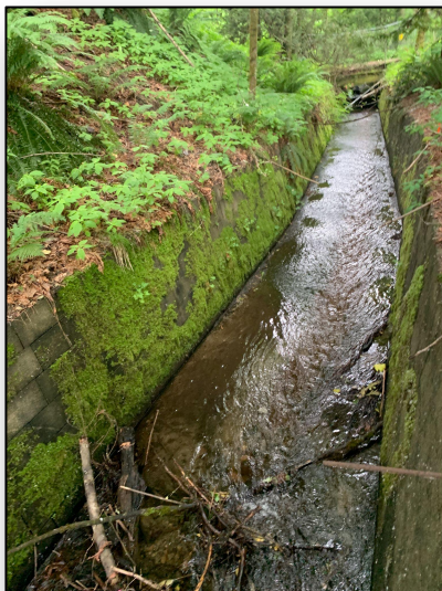
Concrete flume in Bon Accord Creek (before).
