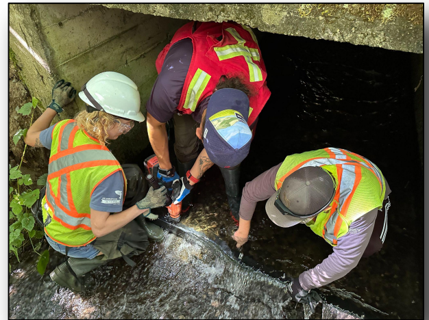
City employees and volunteers working on Bon Accord Creek flume.
