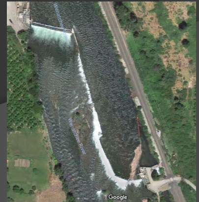
Dryden Dam and Trap
